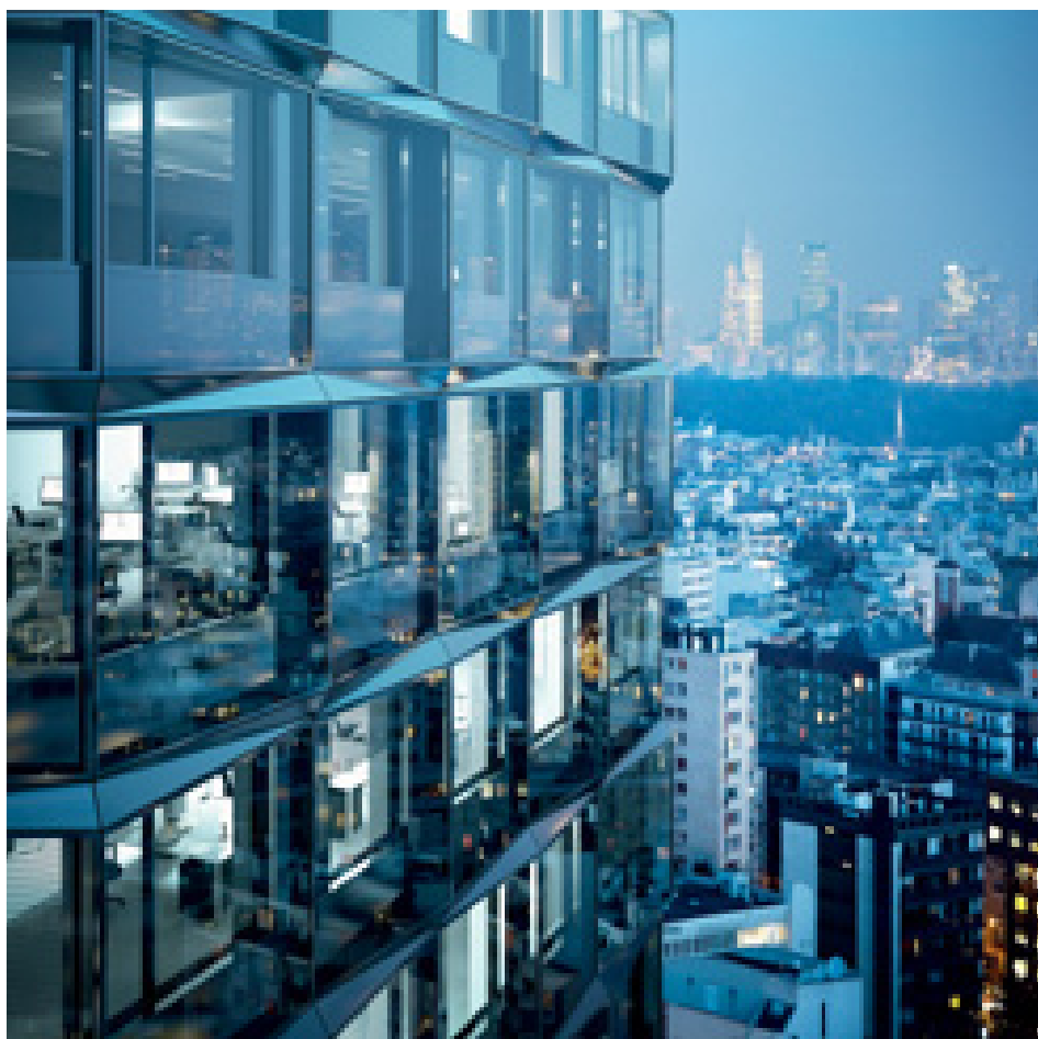
FRANCE: Refurbishment of the Pont du Sèvres towers in Boulogne-Billancourt as part of the Citylights project.
